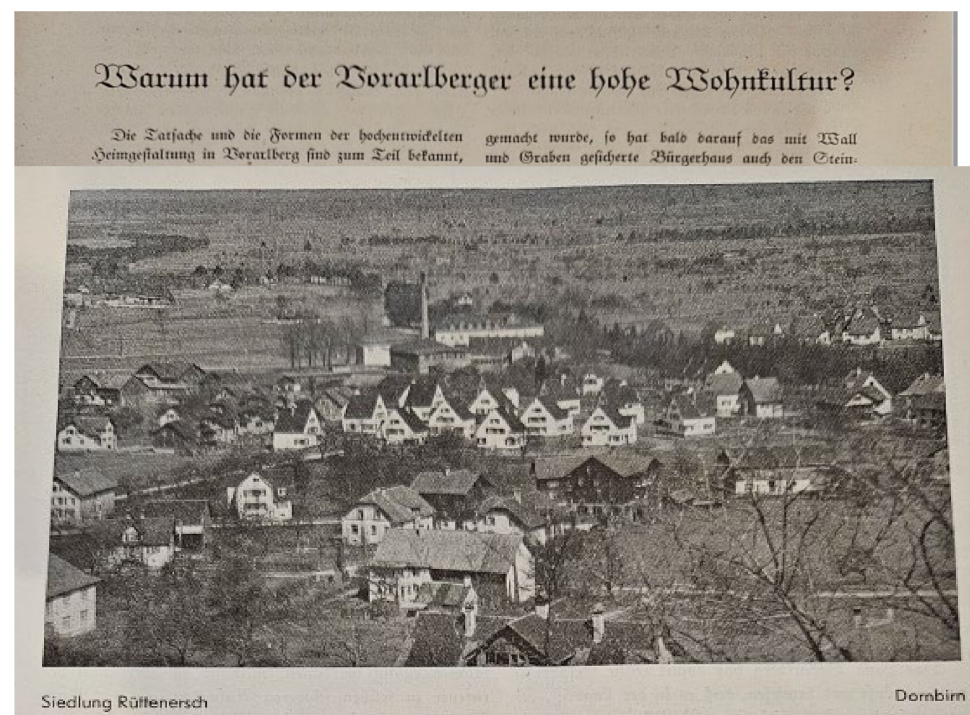
Fig.2: Single-Family-Home-expansion in Vorarlberg, 1931, accompanied by a text praising the high housing culture («Wohnkultur») in Vorarlberg (Wüstenroter Werkschau, 1931)
