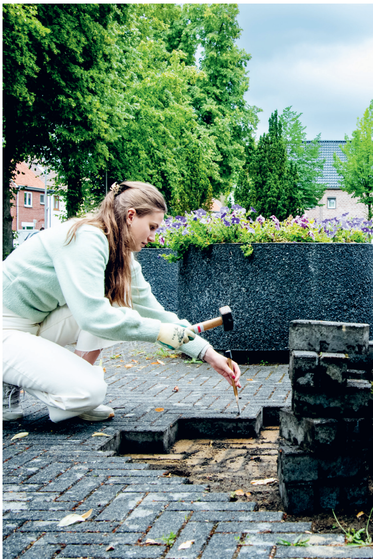
TAKING OUT THE PAVEMENT. Photo: Workshop Team
